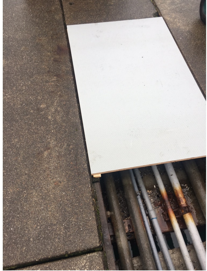
AFTER I-Tech Armor Plated Structural Decking
